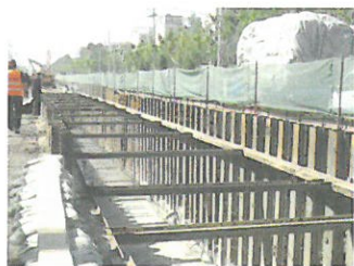
沟槽开挖支撑
